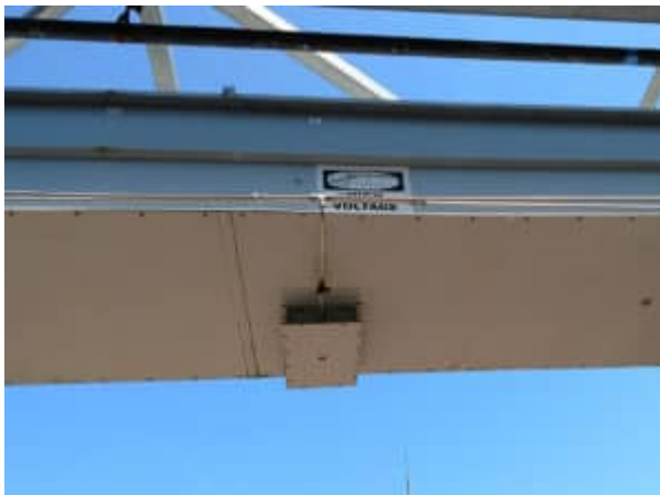
Figure 5: Stainless steel tubing with throttling valve at each heater box
