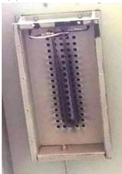
Figure 7: Perforated heater box with air injection tubing penetration
