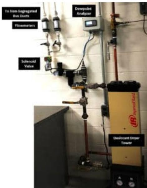
Figure 6: Dry air injection and protection equipment
