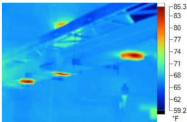
Figure 4: Infrared image of bus duct and space heaters
