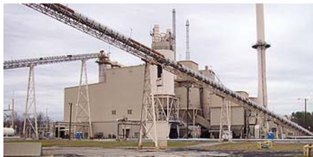
Hopewell Power Station
