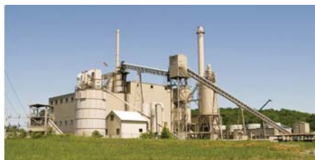
AltaVista Power Station
