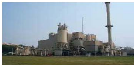
Southampton Power Station
