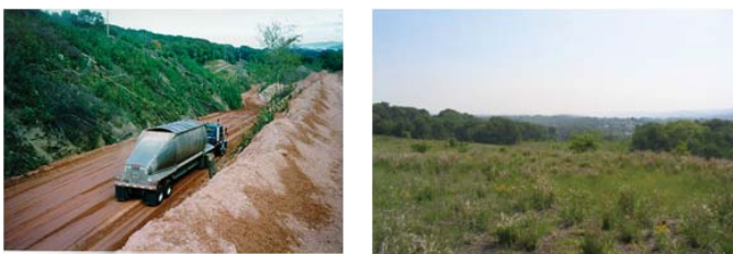
Alden Site – Before and After
