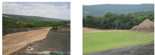
Lommis Site - In Progress
